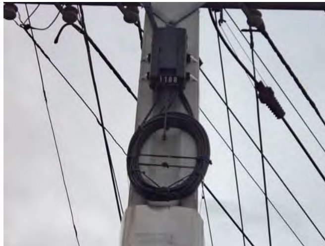
Figure A2.4: Photo showing fibre coil installation
