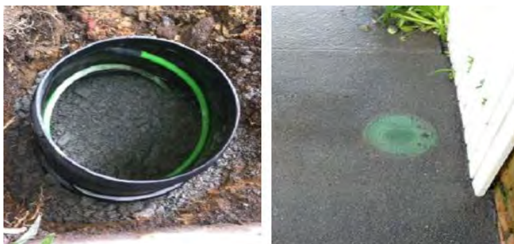
Figure A2.7: Hand hole during and after full installation
